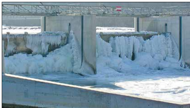
A small frozen hydroelectric power plant in Hronská Dúbrava. The water in small power plants can often freeze and then cause ice floods which endanger the local inhabitants and their homes. Author: Jaroslav Gazdík
